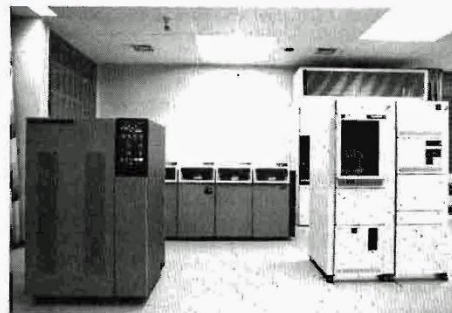
Fig. 3 — Retrieval Centre — Windsor, Victoria.
