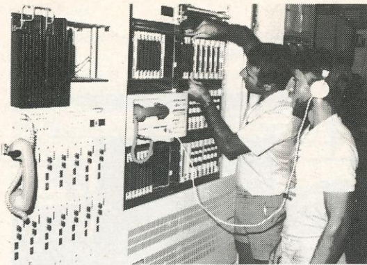
Fig. 21: Installation of the Mt. Magnet Exchange Units
