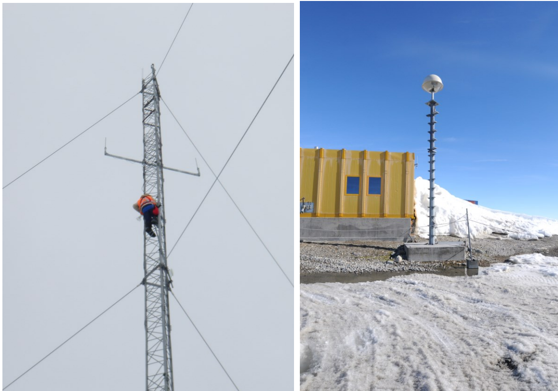
Figure 2 – (a) Technician up a mast at Casey; (b) Davis communications building and mast
