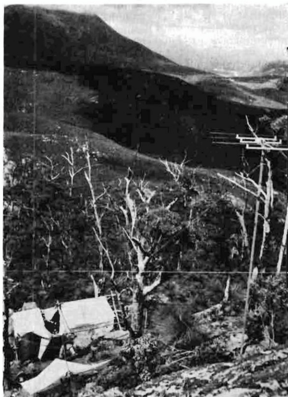
Fig. 22.—Final test station on Mt. Oberon—60 Mc/s aerial is shown pointing to Flinders Island.
