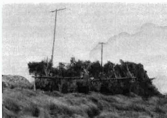
Fig. 28.—Site at Walker's Lookout. Testing installation in early stages. A brushwood windbreak was required as protection against strong winds.
