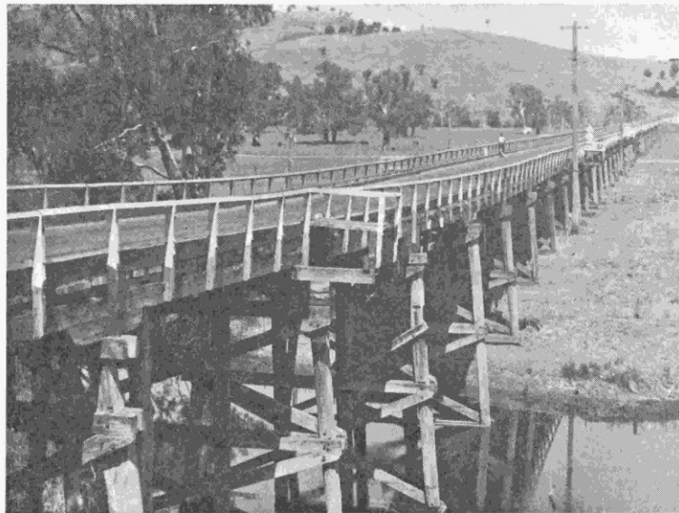
Fig. 6 — Timber Beam Bridge at Gundagai, Southern N.S.W.
