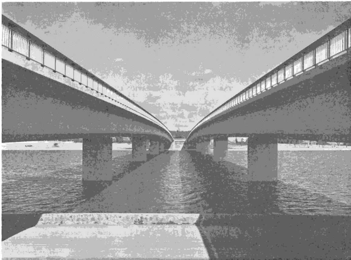
Fig. 8 — Commonwealth Avenue Bridge, Canberra, A.C.T.
