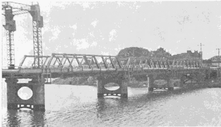
Fig. 5 — Timber Truss Bridge at Murwillumbah, Northern N.S.W.
