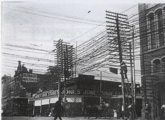
Overhead wires, Perth Town Hall corner, just prior to dismantling, 1915.
