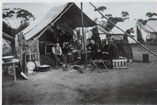
A line party at Zanthus during the 1942 upgrade of the east-west pole route.
